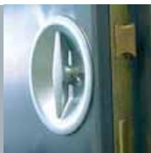
Security interlock on door panel, with key cylinder on floor side and rotating shell on shaft side (as per regulations)
